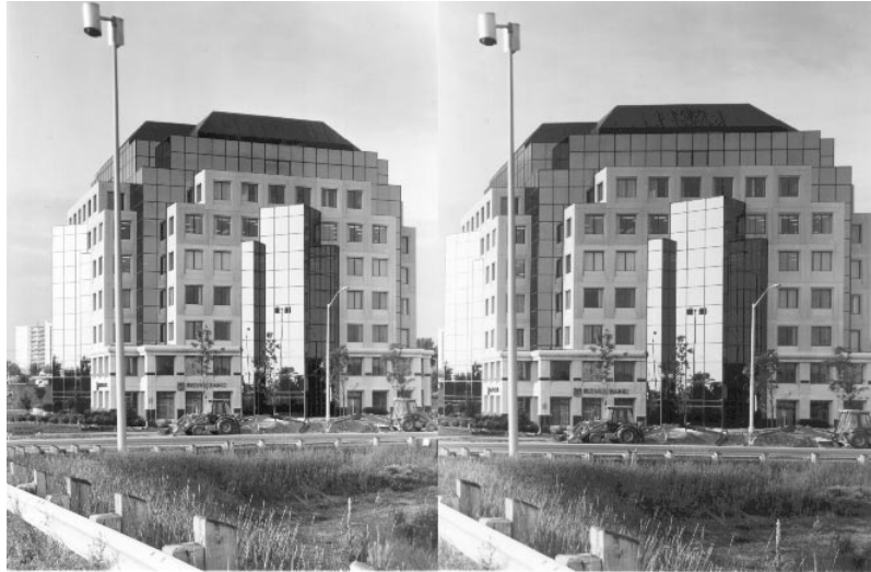
FIGURE 39: a) shows a 'correct' image of a building. Front rise only was used for this photo. In b) the back was swung by almost 38^\circ to give a rather odd and 'incorrect' image. This second photo looks in some ways as though it was taken from a camera position to the photographer's right. But other clues indicate this is not the case: we can see the left side of the building, for example, and we know that most buildings have 90^\circ corners. Swinging the back also stretches the image horizontally.
